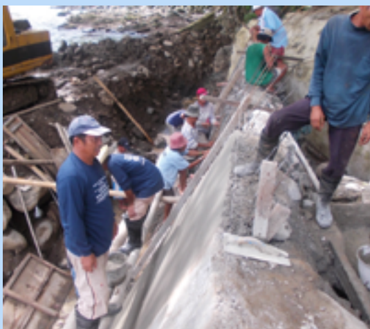
► Figs. 20 & 21. Skilled members of the Mambuaya irrigators' association, under supervision by the National Irrigation Administration, reconstruct the retaining wall and intake box of the river diversion facility.
