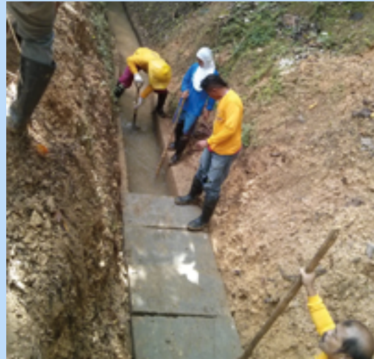
► Fig. 8 & 9. Reinforced concrete covers (above) are cast on-site to protect the newly-unearthed main canal (lef) from future landslides.
