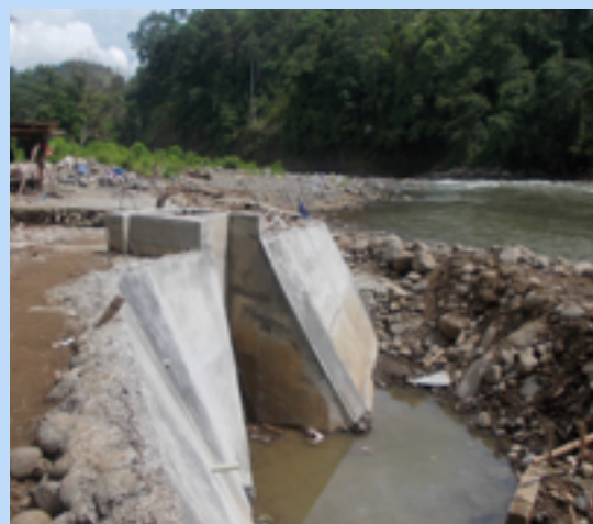
► Figs. 20 & 21. Skilled members of the Mambuaya irrigators' association, under supervision by the National Irrigation Administration, reconstruct the retaining wall and intake box of the river diversion facility.
