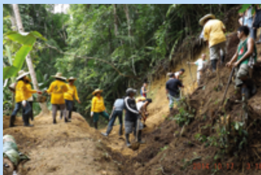
► Figs. 6 & 7. Workers from the irrigators association unearth the main canal that was covered by landslide (above), while the others work on the concrete siphon (left) that serviced farms on the other side of the stream.
