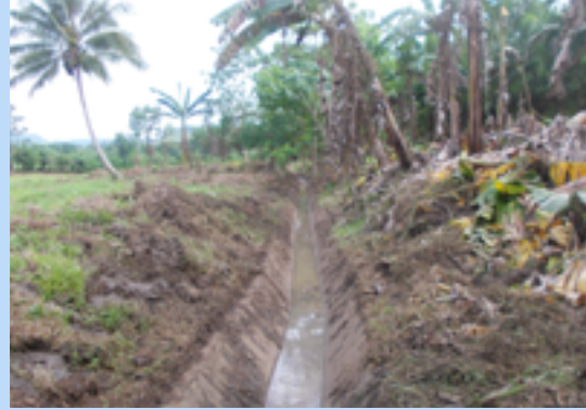
► Figs. 18 & 19. The main canal was also cleared of silt and vegetation and soon irrigation water flowed to the farmlands (right).
