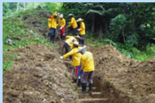
► Figs. 6 & 7. Workers from the irrigators association unearth the main canal that was covered by landslide (above), while the others work on the concrete siphon (left) that serviced farms on the other side of the stream.
