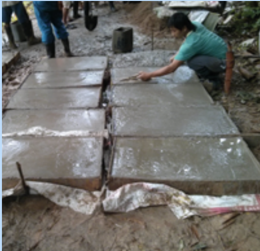
► Fig. 8 & 9. Reinforced concrete covers (above) are cast on-site to protect the newly-unearthed main canal (lef) from future landslides.
