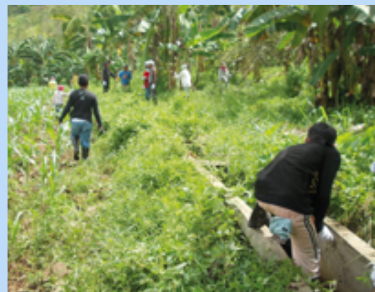
► Figs. 16 & 17. Members of the Mambuaya Irrigators Association clear the lateral canals of vegetation and silt.
