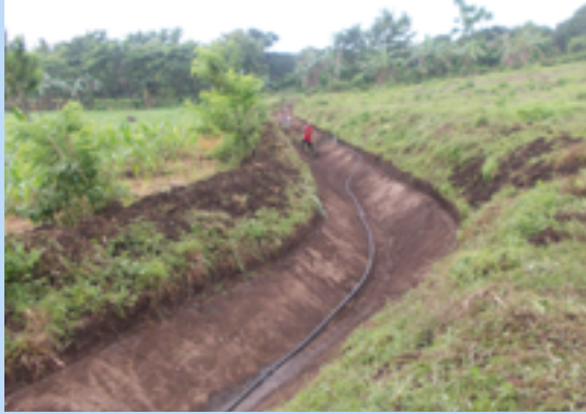
► Figs. 18 & 19. The main canal was also cleared of silt and vegetation and soon irrigation water flowed to the farmlands (right).
