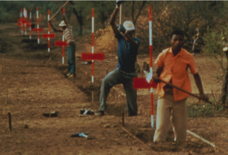
KTC practical training on the setting out of tasks for each worker, Kenya. (Credit: ILO)
