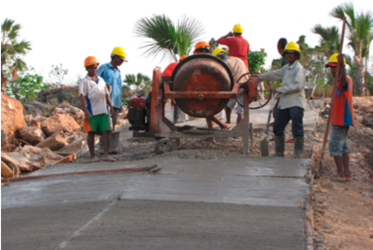
Construction of a concrete road in Timor Leste (Credit: ILO)
