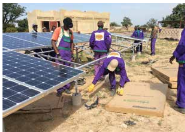
Figure 11. Technician installed mini grid solar plant in Bankoumana
