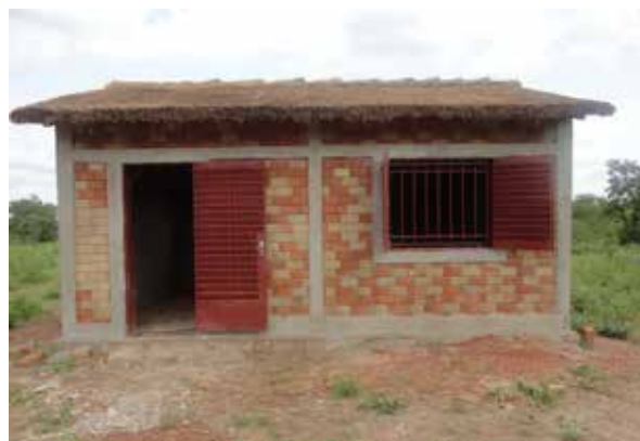
Figure 9. An Ecological Building in Biron, Mali
