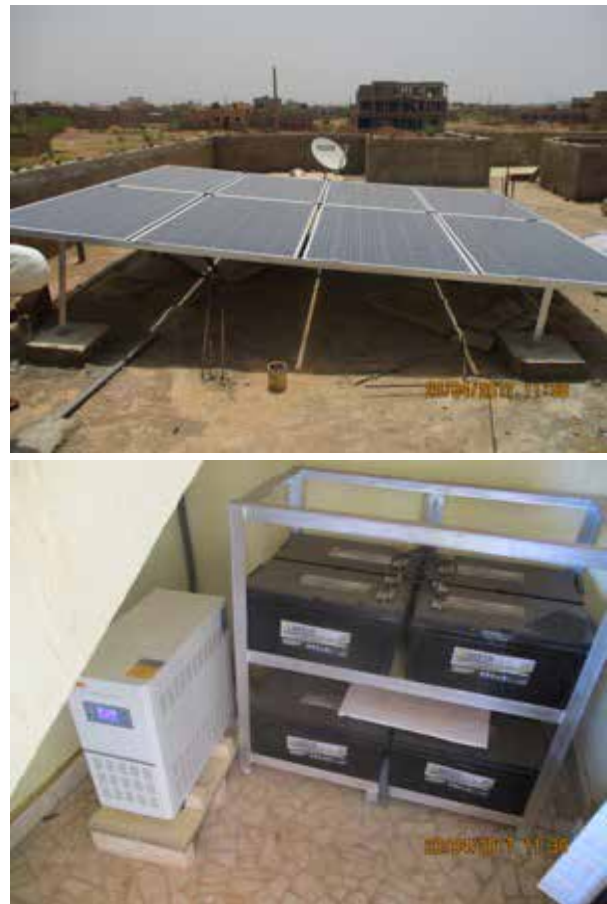
Figure 3. Solar roof installation in a Bamako household
