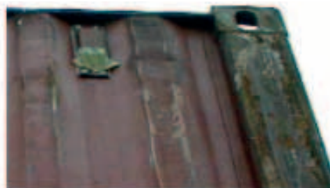
Figure 5.20 – Vent taped over
