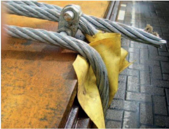
Figure 7.11 – Poor edge protection
