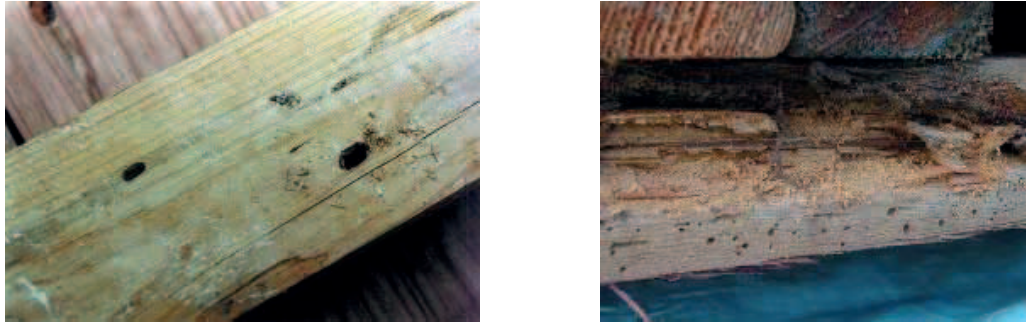
Figure 6.13 – Wood frass from boring insects
