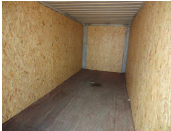
Figure 7.53 – Lining a 40-foot container with chipboard panels
