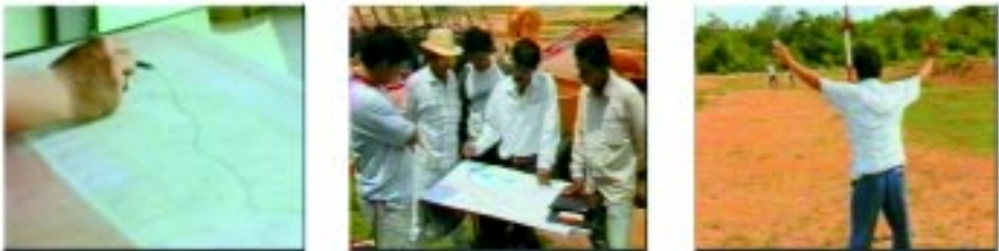
Figure 38: Surveying and setting out of road alignment
