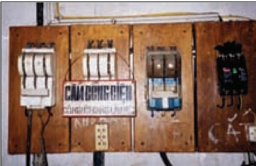
During maintenance, the control should be locked and have a tag "DANGER ! DO NOT OPERATE".
